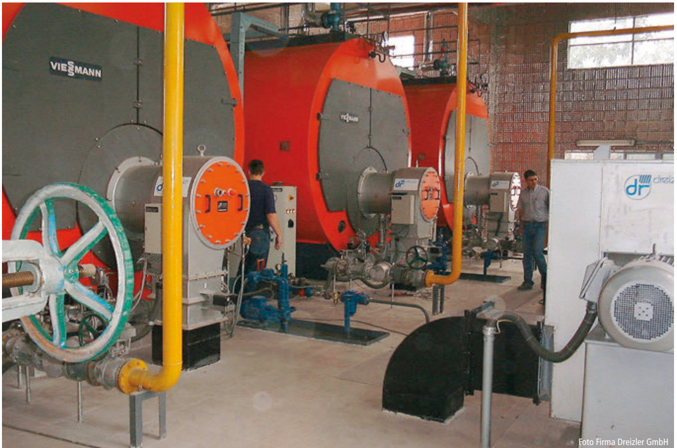
Boiler room of a Chinese airport 25MW, with pressure aggregates from hp-TECHNIK
